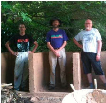
Three men and some brickwork at the new compost bins, Christmas 2010
