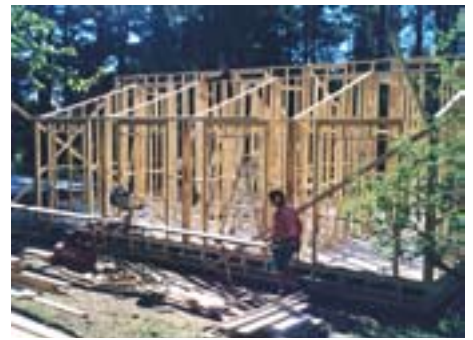
The frame of the new buildings
