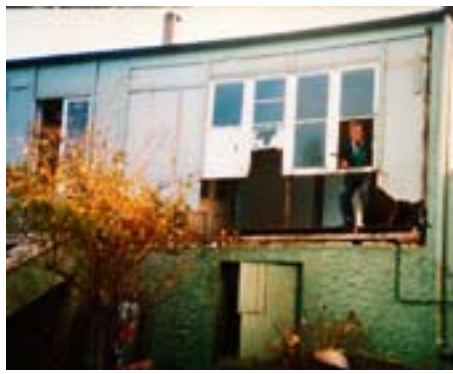
Renovating Sasana House, 1988
