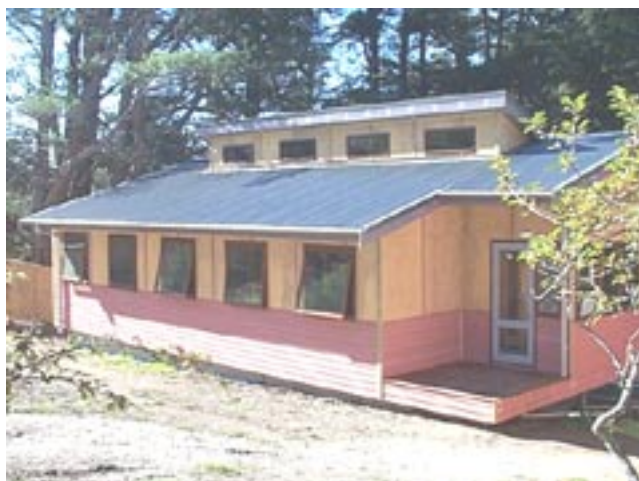
New 9 bedroom accommodation block built entirely with dana . Sadhu, sadhu, sadhu!
