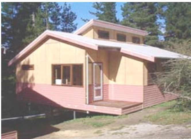
New 7 bedroom accommodation block (also built entirely with dana)
